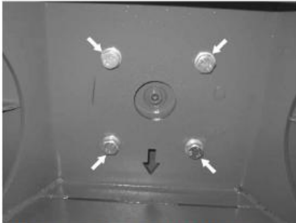
Centre Gearbox Mounting Bolts Location
