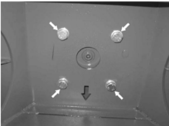
Centre Gearbox Mounting Bolts Location
